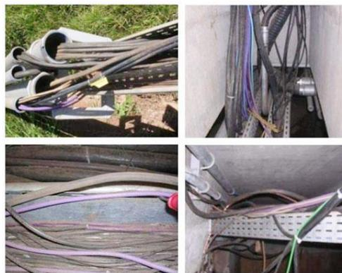
Figure 10 – Examples of Profibus Cable Near to Power Cable
