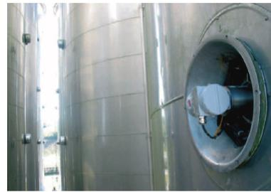
Figure 4: DT3025 Installed on a Fermentation Tank
