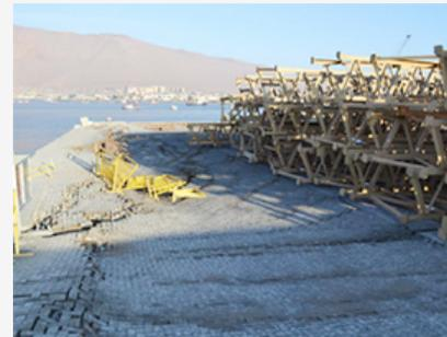
Figure 3: Damage to the north end of Iquique Port Pier 1. Source: Gonzalo A. Montalva and Fernando A. Cerda.
