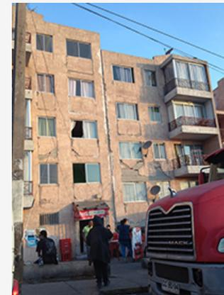
Figure 1: Pounding and infill masonry damage to mid-rise structures. Source: Rene Lagos Engineers.
