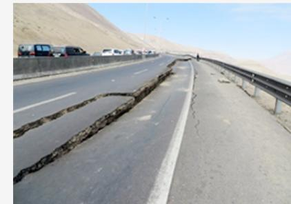
Figure 4: Slope (20°) displacement on Route A16 is 40cm vertical and 10 cm horizontal. Source: Gabriel Candia A.
