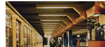
Underground Architecture Berlin
